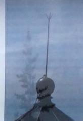
The black ball located directly on top of the lantern roof is called the ventilator ball. The base of this cast iron ball once allowed smoke from the oil lamps to exit the lantern. Brass vents in the walls of the lantern allowed the keeper to regulate the amount of air entering the lantern room.
