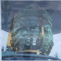
The photo to the left is the latest LED update to the optic. This change took place in 2020, which allowed for the removal of the red shroud around the lens. During daylight you can see the glass lens, but at night when lit, the clear LED lights in the center of the hour-glass shaped optic casts a red light.
